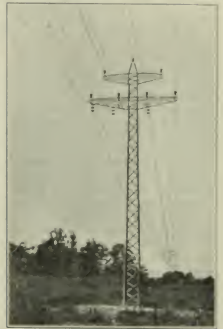
FIG. 15. TOWER USED FOR LINES IN CITIES
